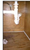
Monitor under a well-sealed sink
